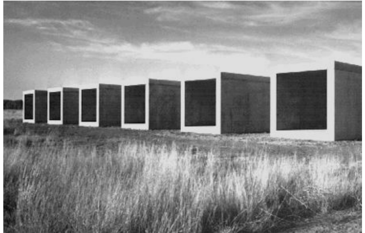
Chinati Foundation, Marfa, Texas Fifteen concrete works.
